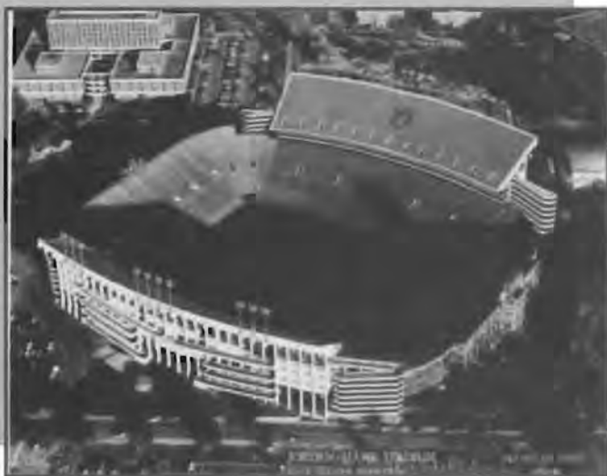
East Stands Addition Jordan Hare Stadium
